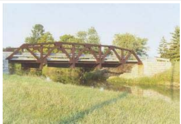
The new Bloody Bridge
